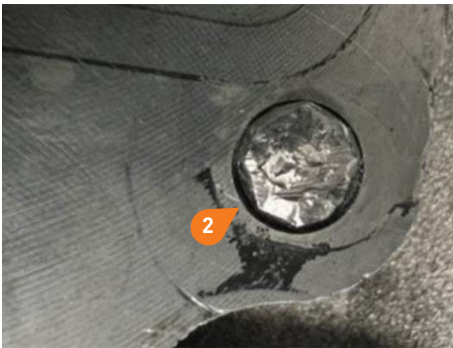
2. The stud / bolt is broken off flush.
